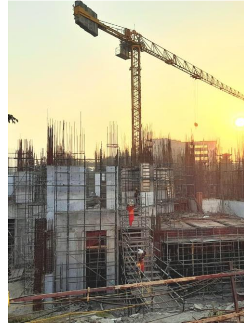
Tower 4 – As on 8 th January 2026 – 1 st floor slab is being casted.
